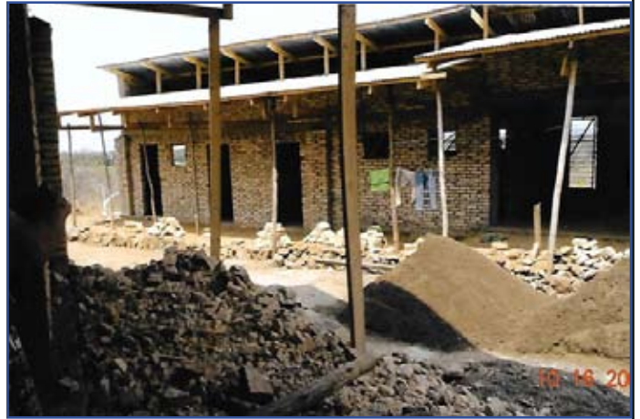
New premises are under construction.
